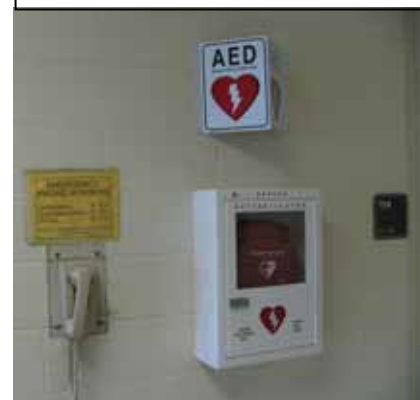
Arlo Wirth Building by room 114
